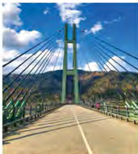
Fig 7.26: Karnali bridge supported by steel rods
