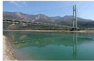
d. Two edges of the bridge
