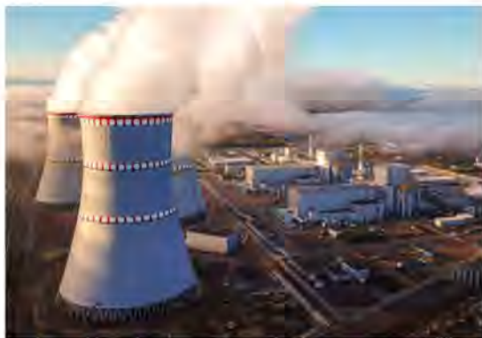
Fig. 1.17 The nuclear power plant in Russia
